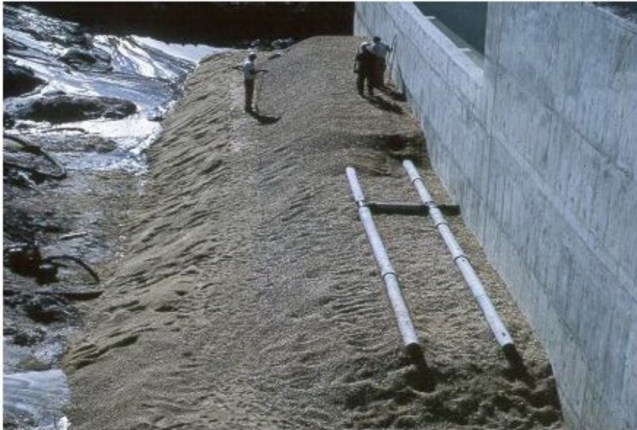
Figure 645K-17 Wall Drain Installation (NRCS-TX)
