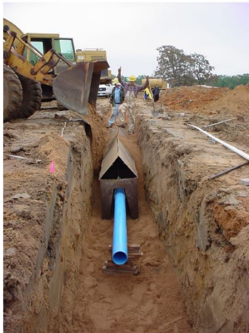
Figure 645K-23 Two-stage Filter Installing the Outer Zone of Fine Materials (NRCS Oklahoma)
