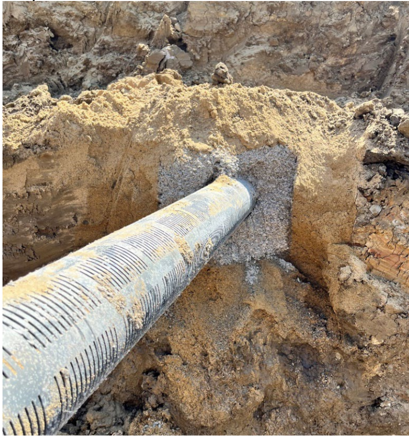
Figure 645K-8 Exposure of a Constructed Toe Drain (NRCS-TX)
