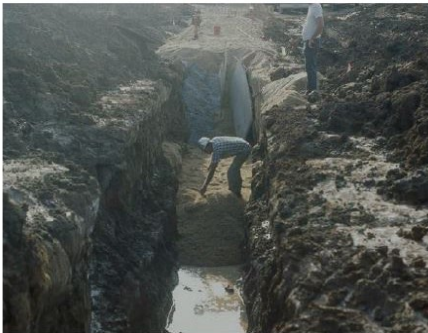
Figure 645K-3 Hazardous Trench Excavation (NRCS-TX)
