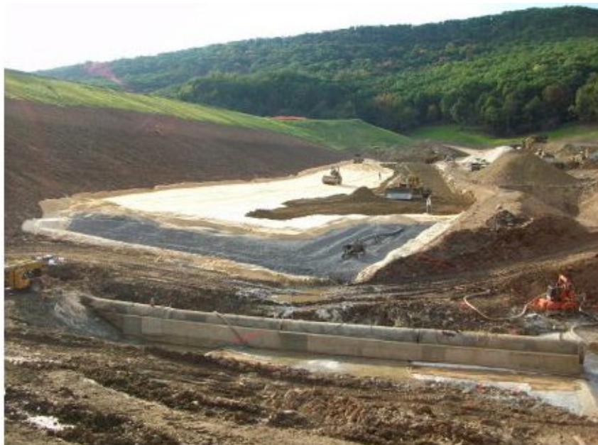
Figure 645K-15 Typical Blanket Drain Installation (NRCS-WV)
