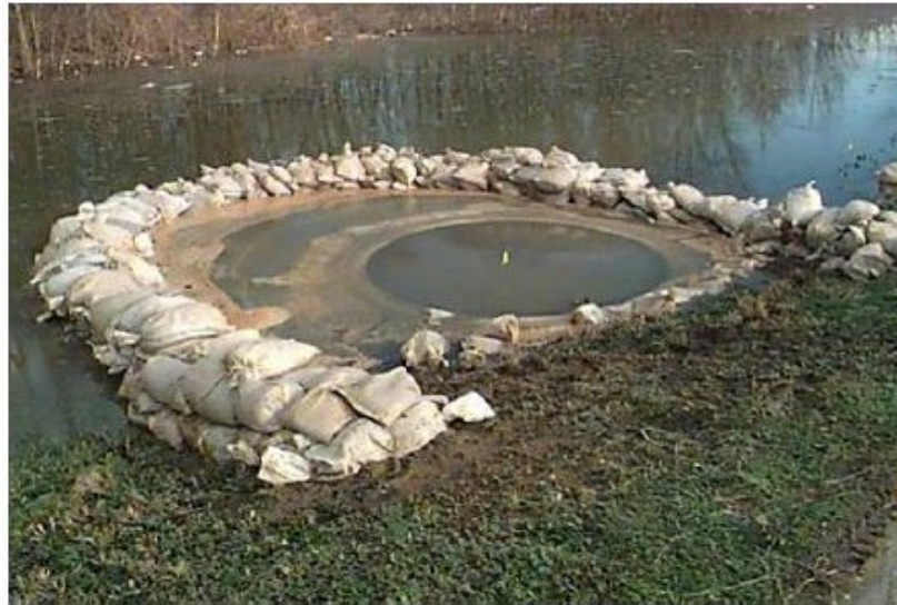
Figure 645K-6 Sand Boil Caused by Uncontrolled Seepage (NRCS-TX)
