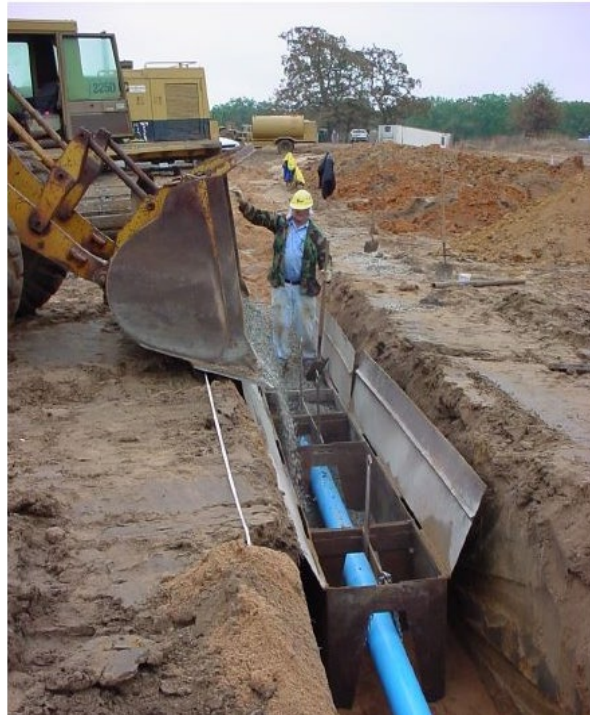
Figure 645K-25 Christmas Tree Method of Installing Filter Material
