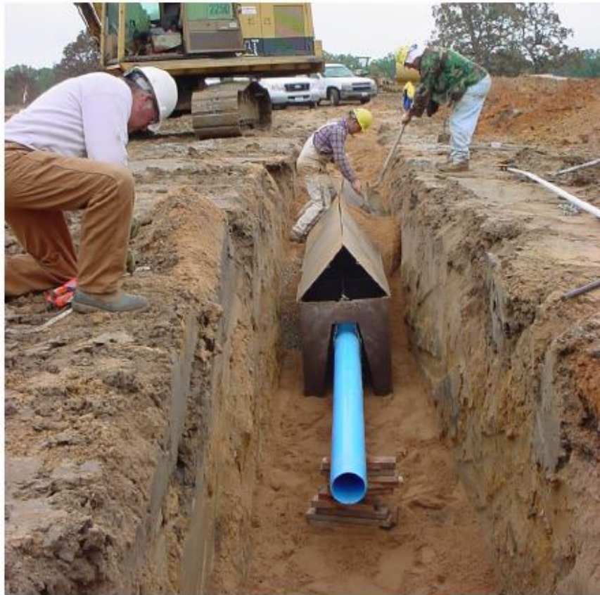
Figure 645K-4 Proper Trench Excavation (NRCS-OK)
