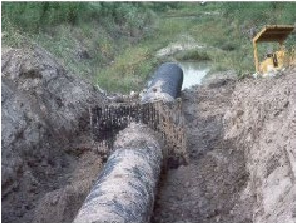
Figure 645K-10 Anti-seep Collar (NRCS-TX)
