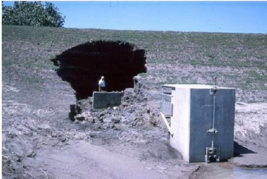
Figure 645K-5 Embankment Failure Caused by Seepage along Principal Spillway (NRCS-TX)
