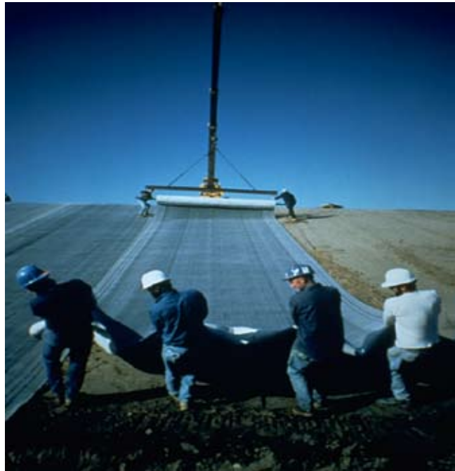
Figure 10E-7 Stationary pull
