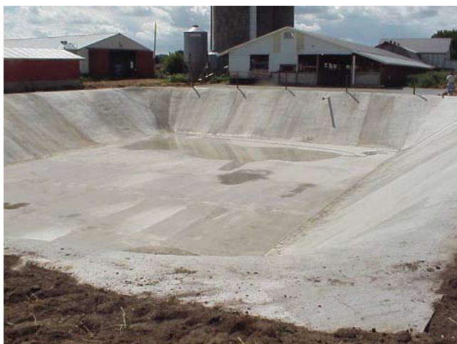
Figure 10D-3 Excavated animal waste storage pond with concrete liner ( Photo credit NRCS )
