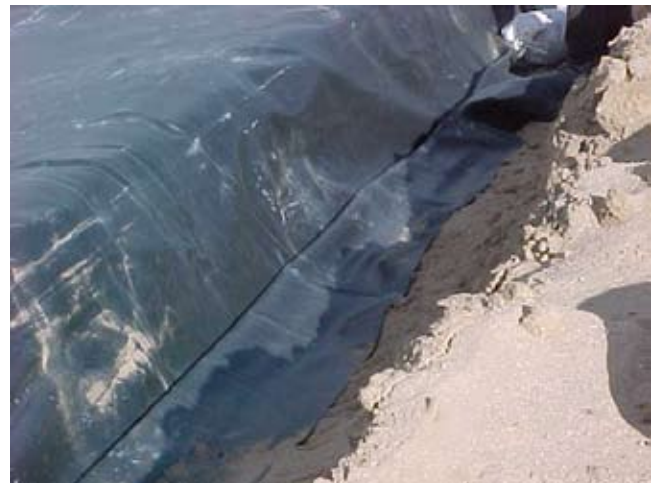
Figure 10E-12 Anchor trench details (Source: Poly-Flex, Inc., 1995)
