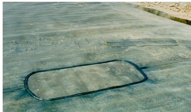
Figure 10E-30 Liner repair
