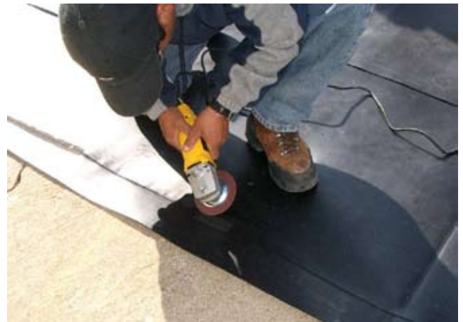
Figure 10E-16 Grinding for an extrusion weld
