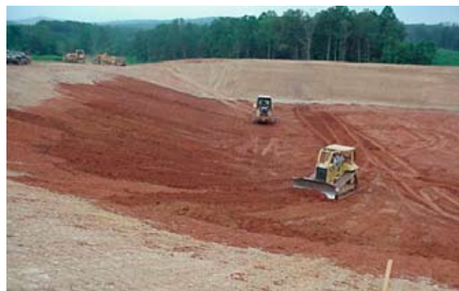
Figure 10D–11 Bathtub construction of clay liner ( photo courtesy of NRCS Virginia (top) and NRCS Nebraska (bottom) )
