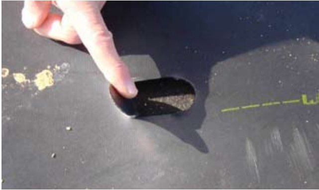
Figure 10E-28 Uncovered liner vent
