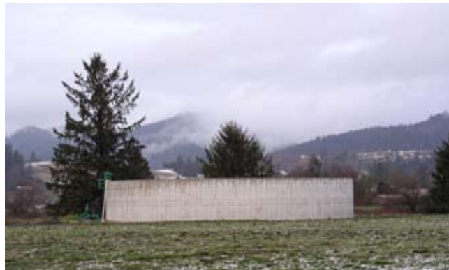
Figure 10D-4 Aboveground storage tank for animal waste ( Photo credit Mitch Cummings, Oregon NRCS )
