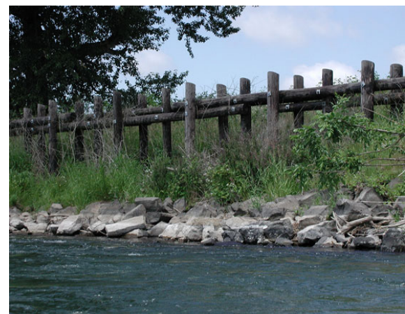
Figure 610–10 Rock and timber revetment on the Willamette River, Oregon (photo courtesy Kathryn Boyer, USDA NRCS)
