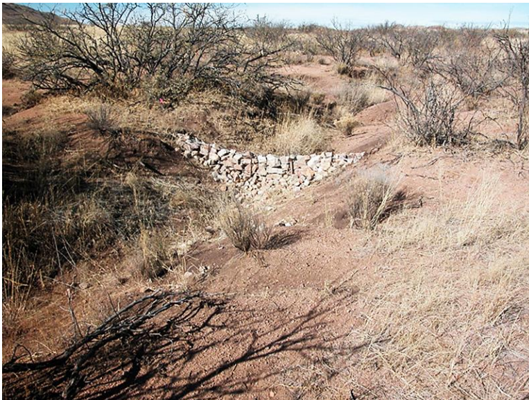
Figure D-6. Rock gully plug in southern Arizona used to retard overland flow and trap sediment behind, reducing further downstream erosion through reduction in runoff velocity.
