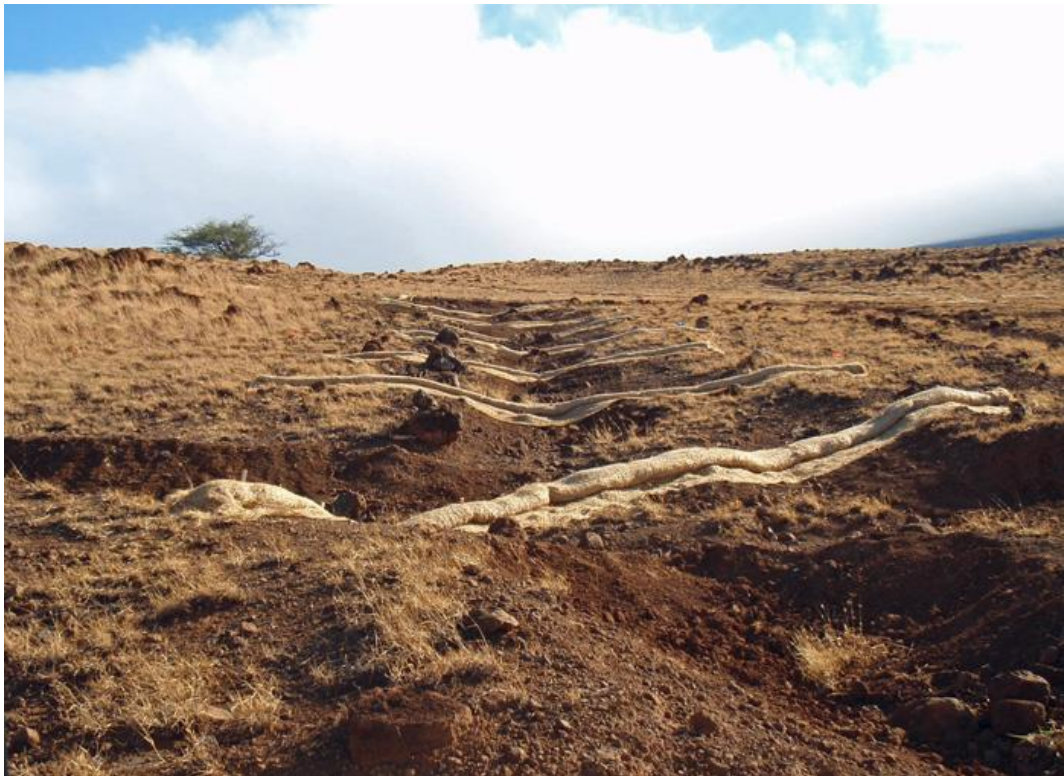
Figure iii. Soil erosion control using straw-filled wattles in Pelekane Bay, Hawaii.
