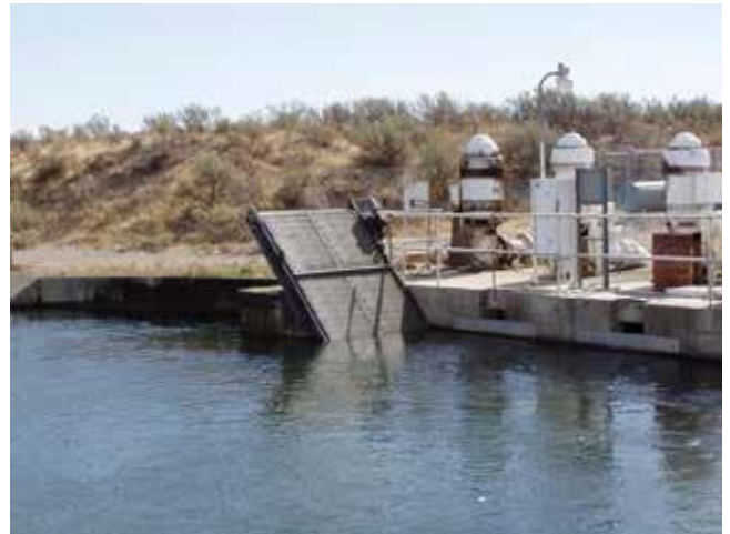
Figure 8B–2 Slanted screen with moving brush Ontario, OR
