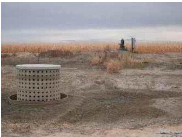
Figure 8B–9 Perforated concrete drainage pipe used as a coarse screen Ft. Morgan, CO
