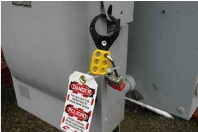
Figure 8–92 Lockout and tagging of power switch
