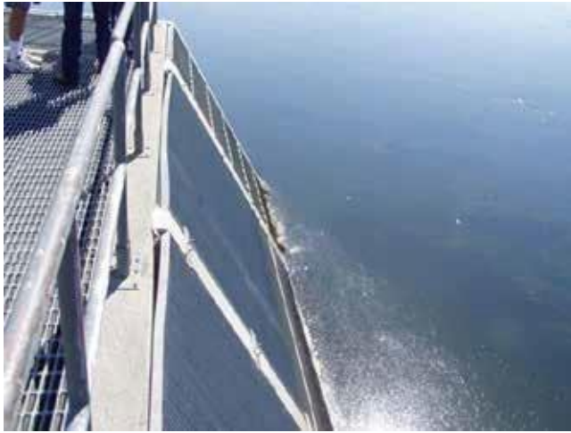
Figure 8B-6 Slanted stationary screen Richland, WA
