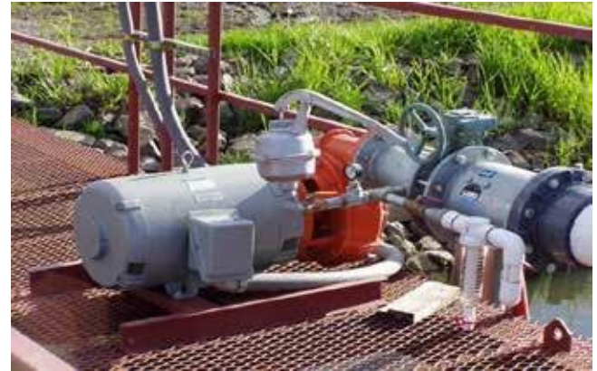
Figure 8–32 Priming with foot valve and hand primer, blueberry farm near Fargo Lake, WA
