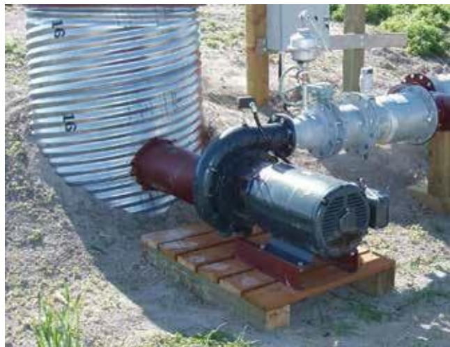
Figure 8-15 Horizontal centrifugal pump for surface or pit installation
