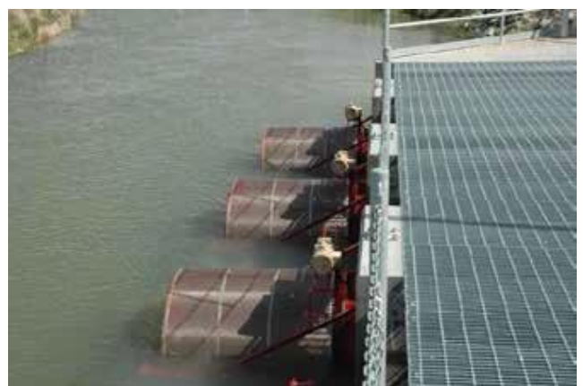
Figure 8B–3 Bank of rotating circular screens with internal sprays Farson, WY
