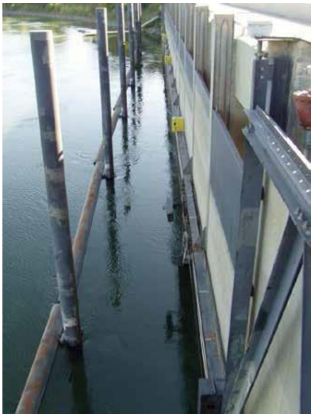
Figure 8B-5 Vertical stationary screen Colusa, CA
