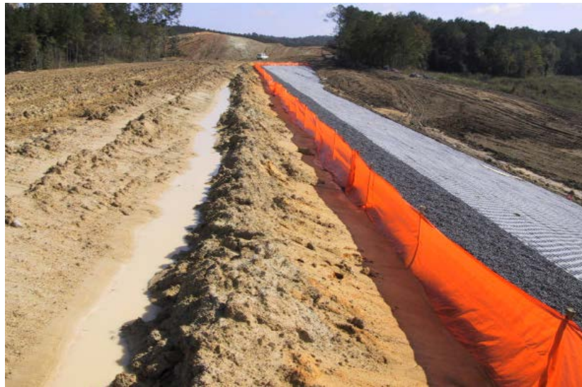
Figure 34: Top of ACB Installation During Dam Construction (photograph perspective is looking from top to blocks at right)
