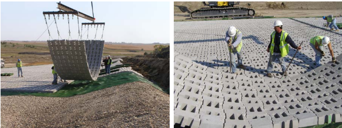
Figure 45: ACB Installation, NRCS-North Dakota
