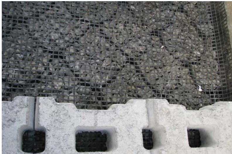
Figure 26: Three Dimensionally Confined Drainage Layer Used to Increase Stability of ACB Units Under Hydraulic Jump Conditions
