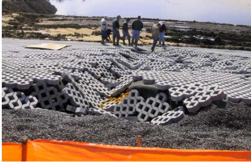
Figure 37: Eroded Soil From Under Geotextile Deposited Further Down the Slope (photo perspective is looking downslope)
