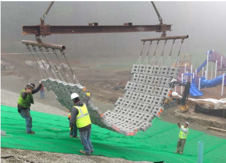
Figure 33: Typical ACB Installation (green material in photograph is the geogrid confinement)
