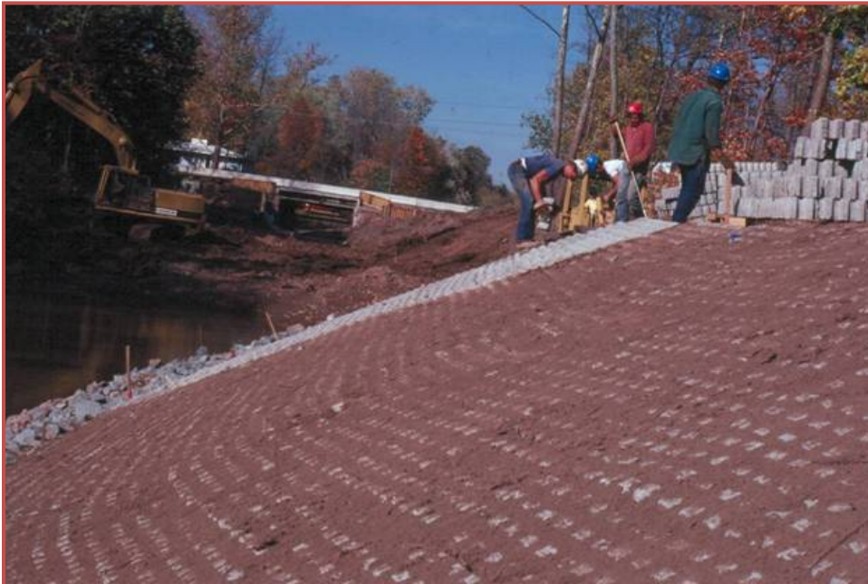
Figure 43: Soil Added to an ACB Channel Lining
