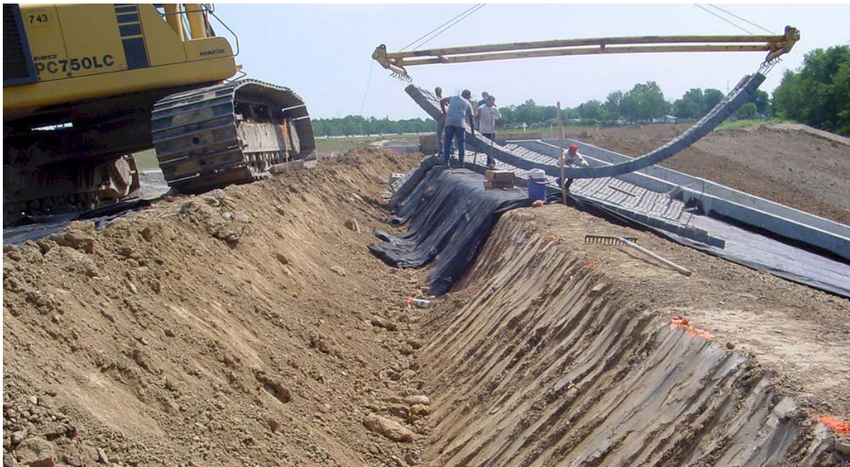
Figure 42. Termination of ACBs at Concrete Cutoff Wall (N.T.S.)
