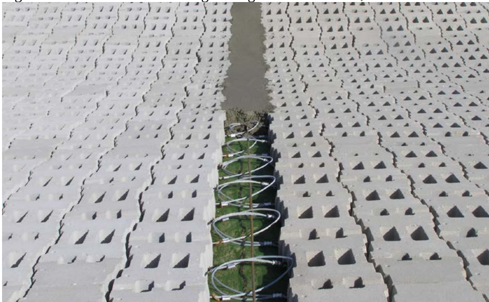
Figure 46: Grouted Mats Abutting During ACB installation, NRCS-ND
