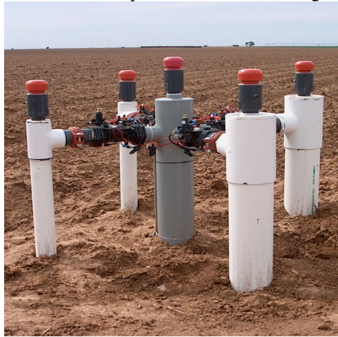
Figure 4-39 Air valve placement on a microirrigation manifold
