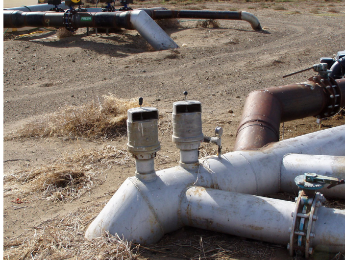
Figure 4-34: Continuous acting air valve
