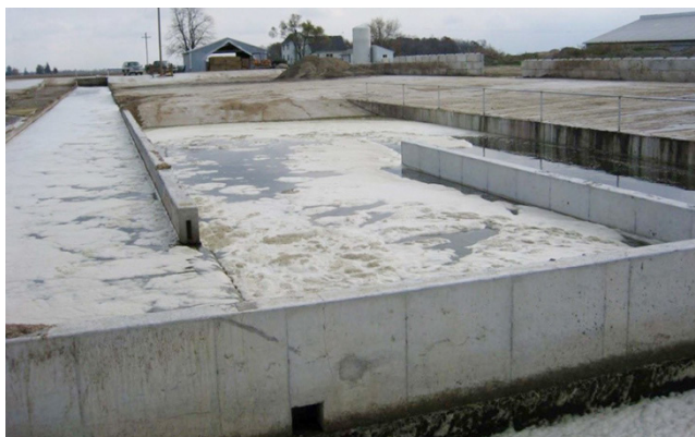
Figure 4–49 Effluent from a sand lane falling directly into a settling basin (Holmes 2010)
