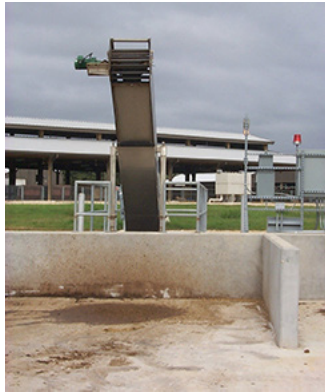
Figure 4–8 An in-channel flighted conveyor separator and solids stacking area (Mukhtar et al. 1999)
