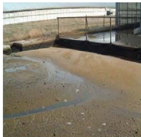
Figure 4-50 Sand trap positioned on the end of a flushed, two-row freestall barn (Wisconsin University, Cooperative Extension & Kansas State University, Cooperative Extension, Harner 2009).
