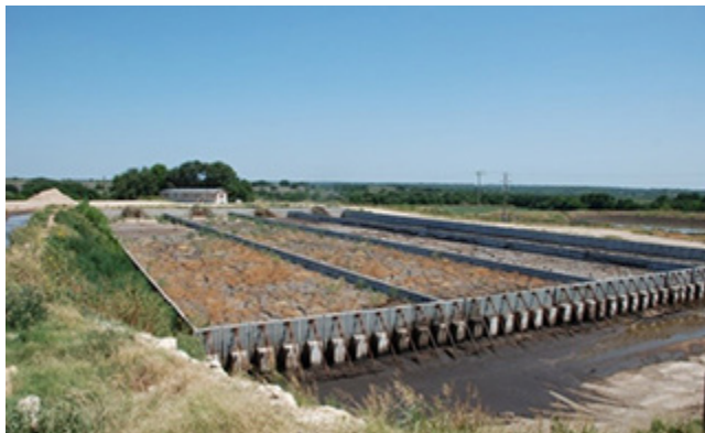
Figure 4–62 A large, multichambered primary weeping wall settling basin by Mukhtar et al. (2011)
