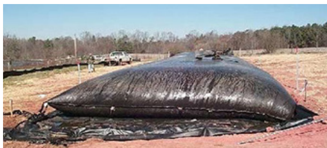
(a) Geotextile tube used in Georgia without chemical enhancement (45 ft circumference × 100 ft long).
