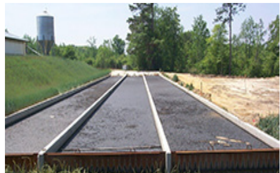
Figure 4–3 Settling basins arranged in parallel to provide primary treatment for liquid manure (Mukhtar et al. 1999)
