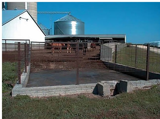
Figure 4–1 Settling basin to provide primary treatment for feedlot runoff (Iowa State University Extension)
