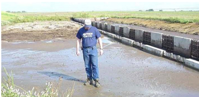
Figure 4–60 Full settling chamber with sand near the fill end (beneath the dairy producer and accumulated dairy solids at the back) (Fulhage 2003)
