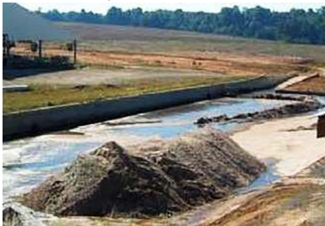
Figure 4–52 Recovered sand storage and concrete access ramp used with a sand beach (Kansas State University Cooperative Extension, Harner 2009)
