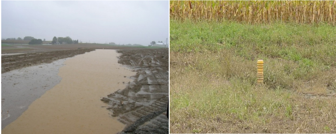
Figure 8-44: Underground Outlet System Storage Pool Figure 8-45: Underground Outlet System Inlet
