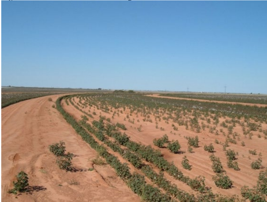
Figure 8-35: Terraces with Level Alignment
