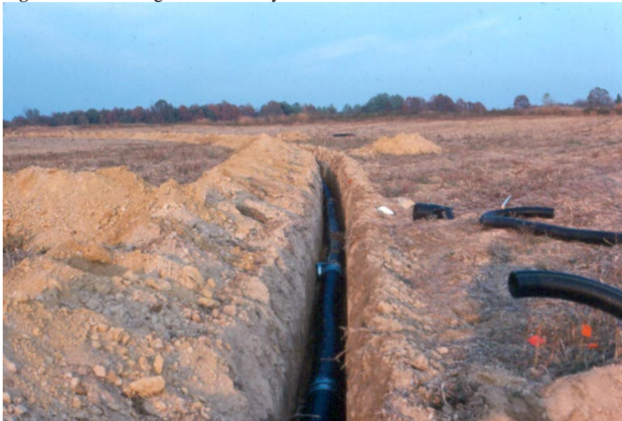
Figure 8-46: Underground Outlet System Conduit
