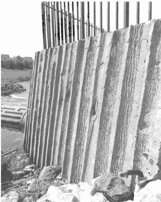
Figure 11-87: A Pond Structure with Textured Concrete Surfaces
