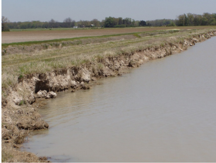
Figure 11-69: Bank Erosion Form Wave Action
