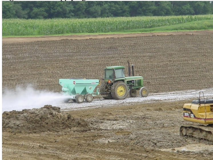
Figure 11-82: Applying Soda Ash to the Pond Bottom
