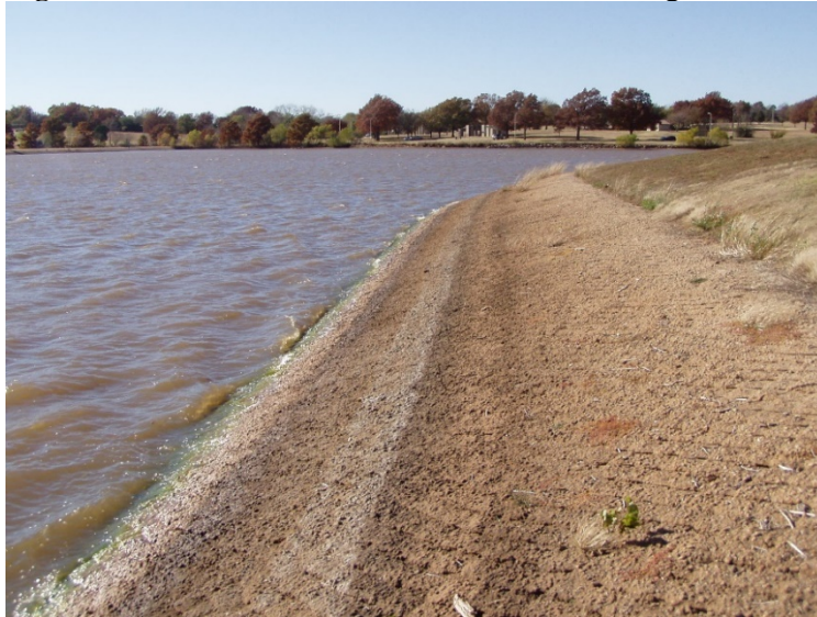
Figure 11-70: Soil Cement Mat Used to Protect Against Wave Action
