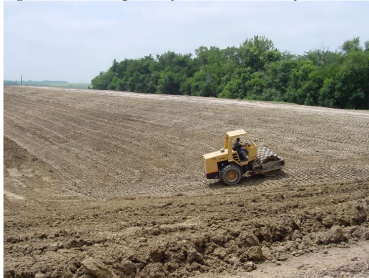
Figure 11-81: Using a Sheepsfoot Roller to Compact the Pond Surface
