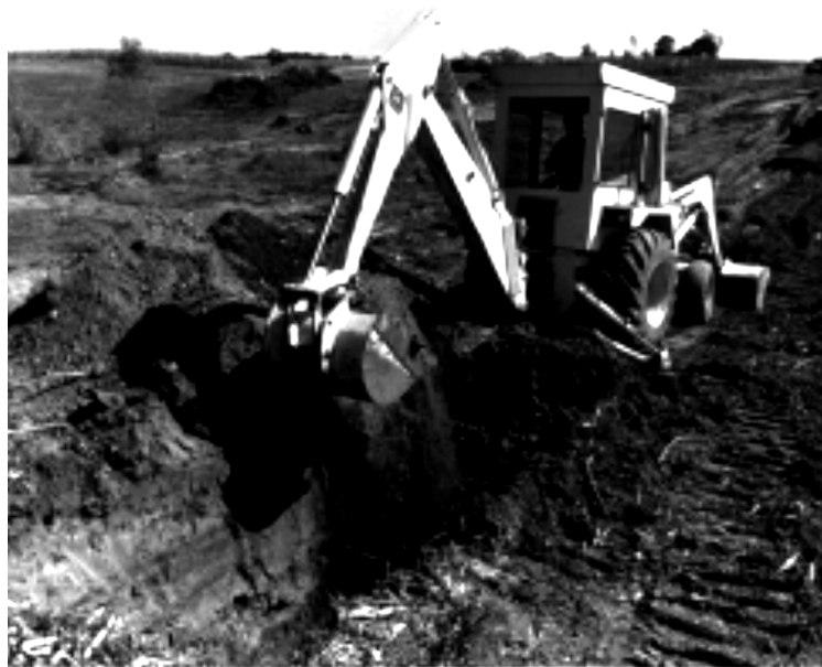
Figure 11-47: A Core Trench is Cut Along the Centerline of a Dam
