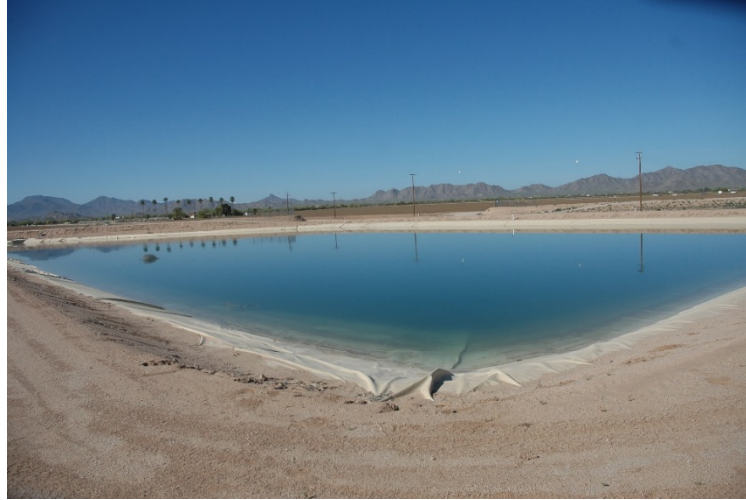
Figure 11-83: An Arizona Pond with a Flexible Membrane Liner
