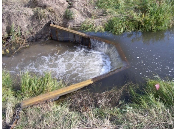
Figure 13-40: Sheet Pipe Vortex Weir
