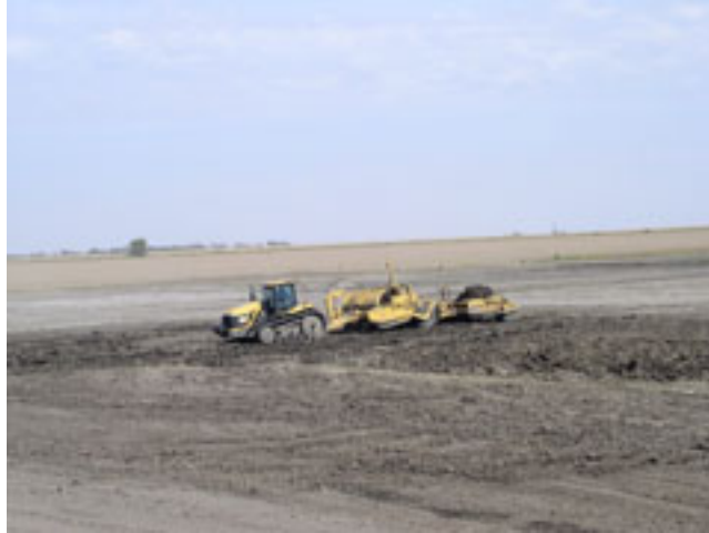
Figure 13-67: Wetland construction often requires low ground pressure equipment.
