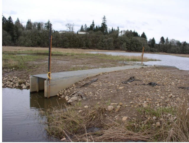
Figure 13-49: Fish Passage between a Stream and a Wetland
