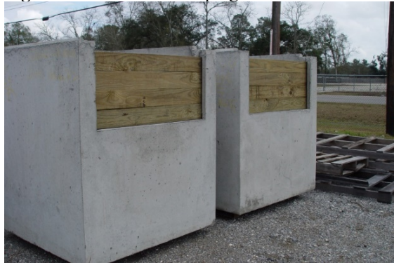
Figure 13-42: Precast Stoplog Structures
