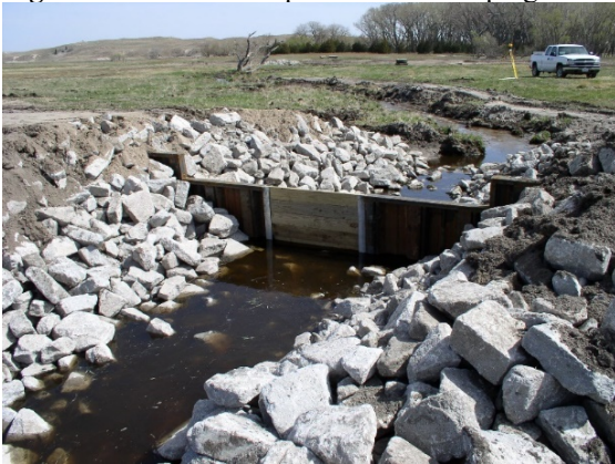
Figure 13-41: Sheet Pipe Weir with Stoplogs
