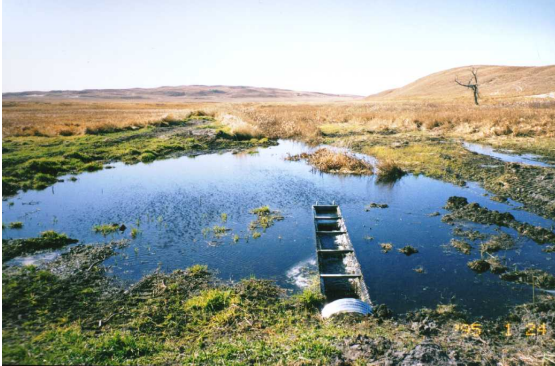
Figure 13-39: Cut Pipe Culvert
