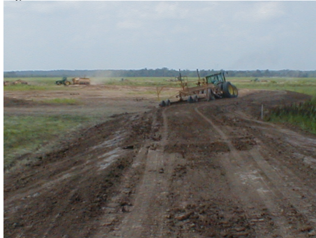
Figure 13-33: Dike for Internal Water Control
