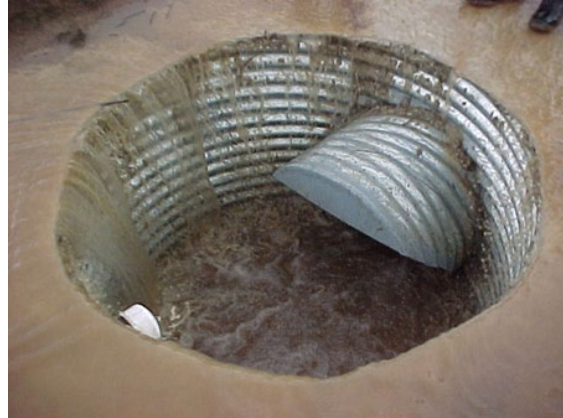
Figure 13-46: Riser with Canopy Barrel Inlet
