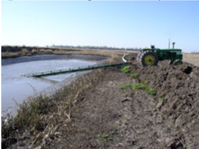
Figure 13-66: Dewatering a Pit to be filled as part of a Restoration
