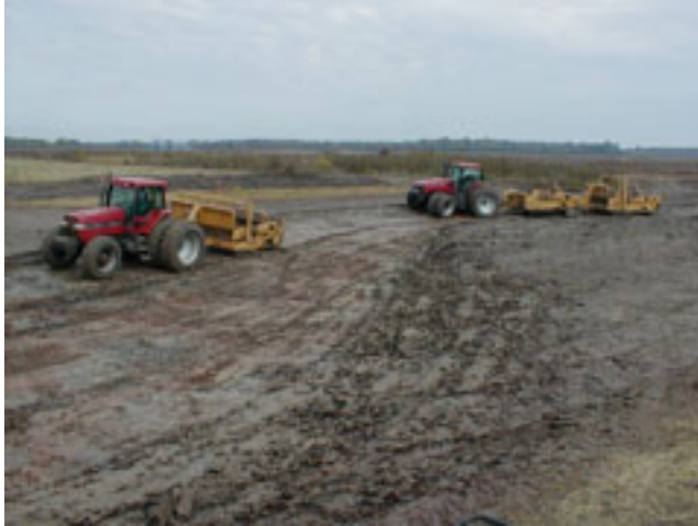
Figure 13-65: Construction in a Riverine Wetland Project
