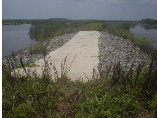
Figure 13-48. Armoring Auxiliary Spillway with Concrete and Riprap
