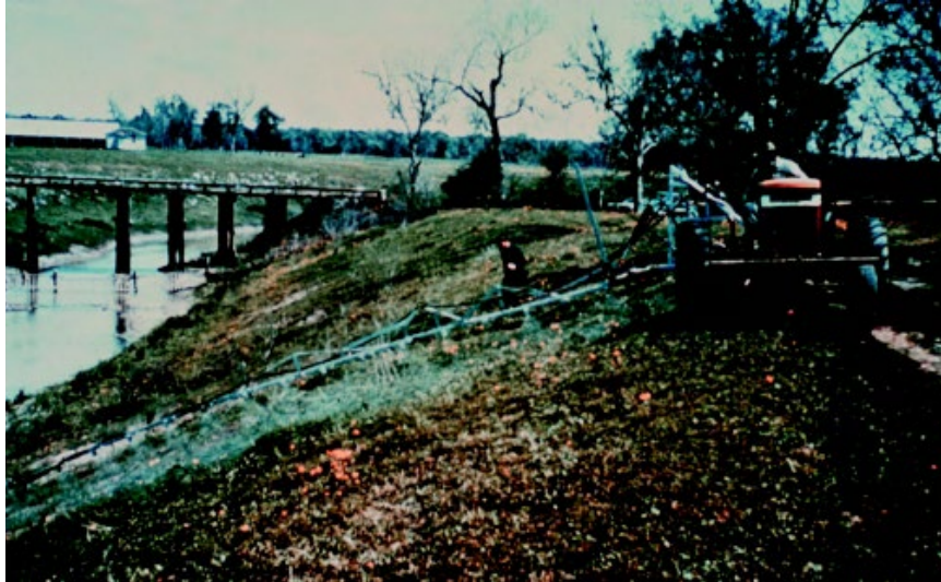
Figure 14-28: Application of Chemicals for Side Slope Weed Control
