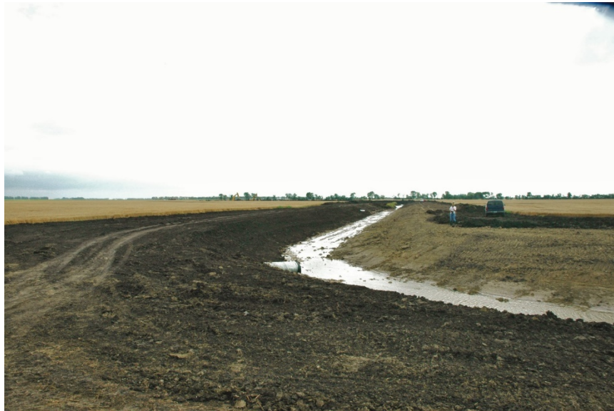
Figure 14-25: Main Drain with Spoil Banks Spread
