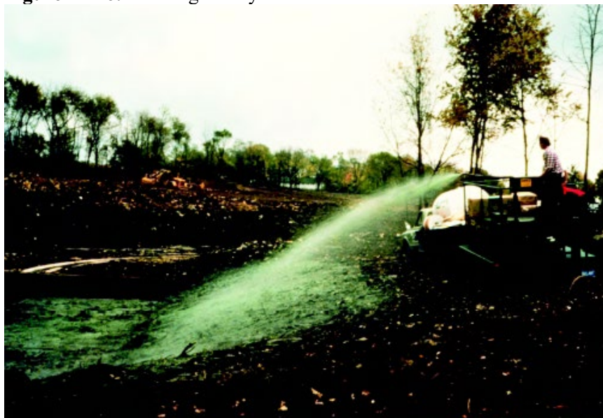
Figure 14-26: Seeding Newly Constructed Drain
