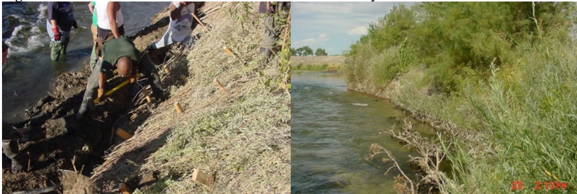
Figure 16-2: Brush Mattress. Under construction and after 2 years.
