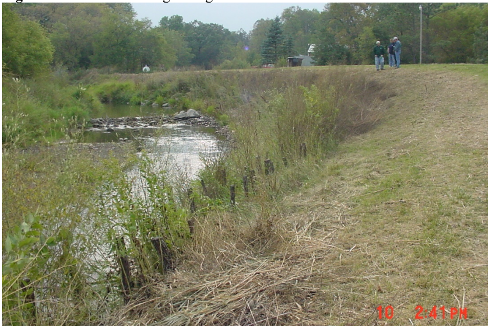
Figure 16-9: Live Stakes growing on stream bank one season after installation.
