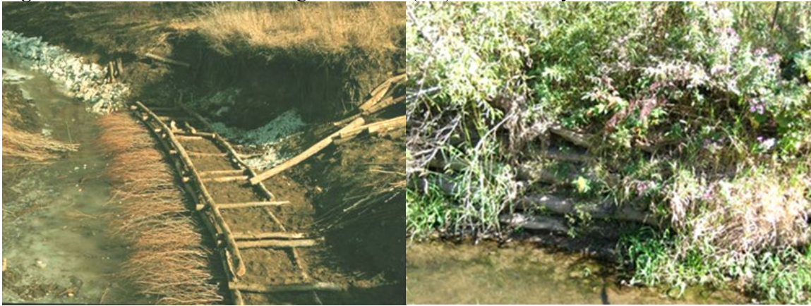
Figure 16-13: Live Cribwall during Installation (left) and after 10 years
