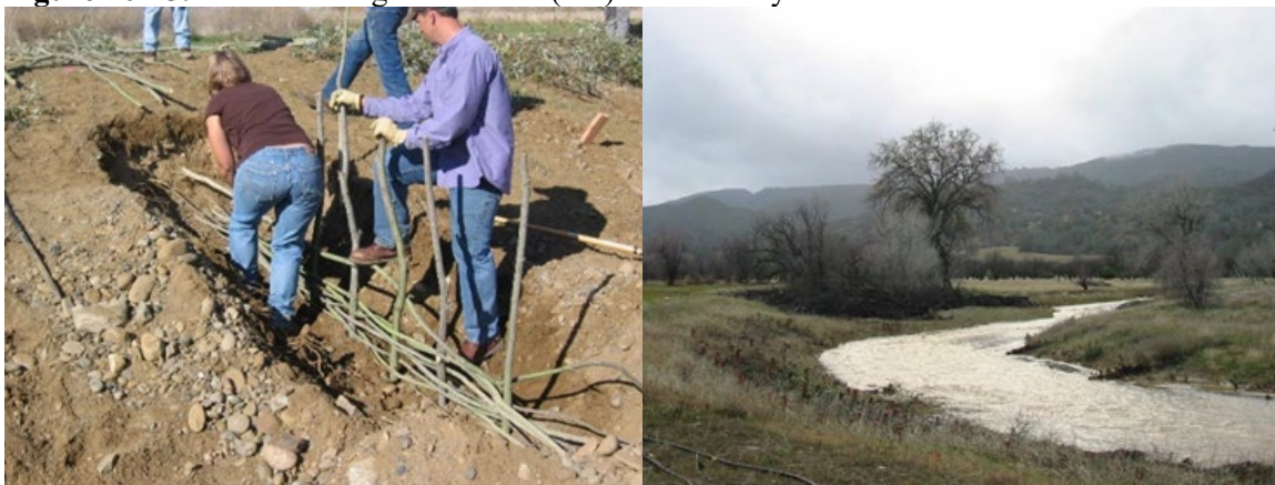
Figure 16-15: Wattle during Installation (left) and after 2 years
