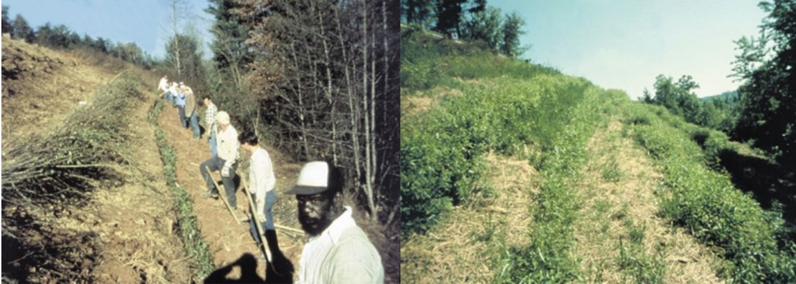
Figure 18-10: Example Live Fascine System Installation and 3 Months After Installation
