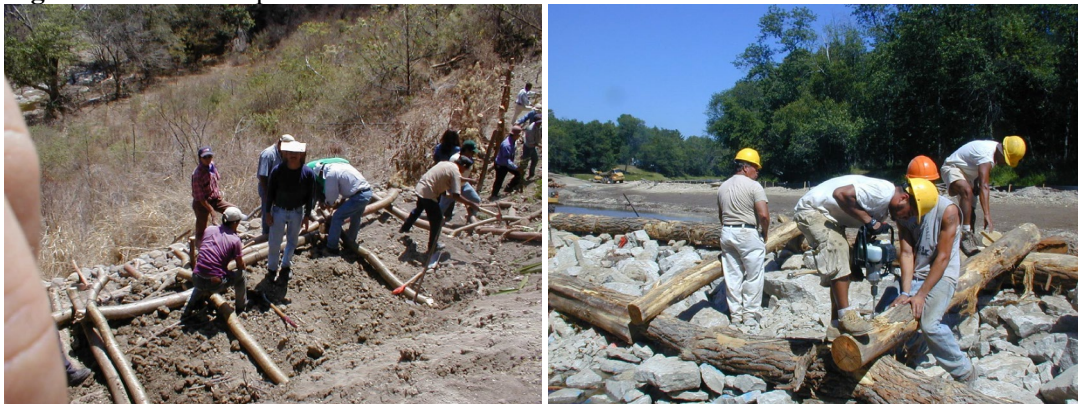
Figure 18-18: Example Live Cribwall Installation
