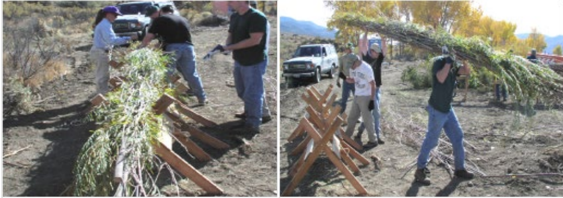
Figure 18-9: Fabrication of a Live Fascine Bundle
