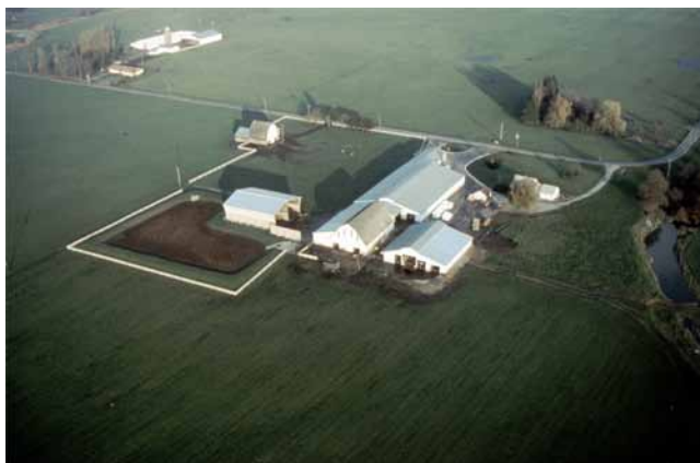
Figure 8–17 Farmstead buildings effectively block views to a waste storage pond.
