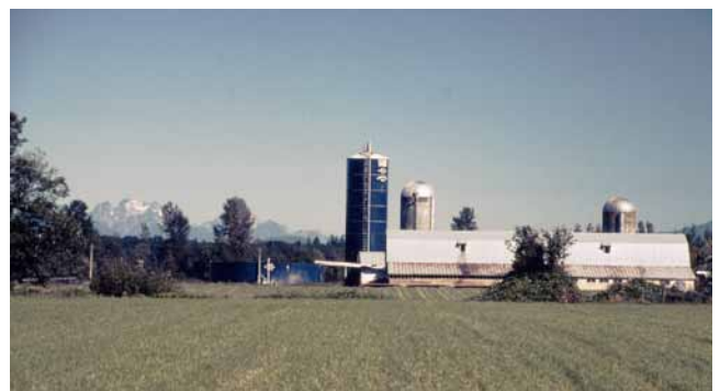
Figure 8–10 An aboveground storage tank is inconspicuous on this highly scenic landscape due to careful design, siting, and color.
