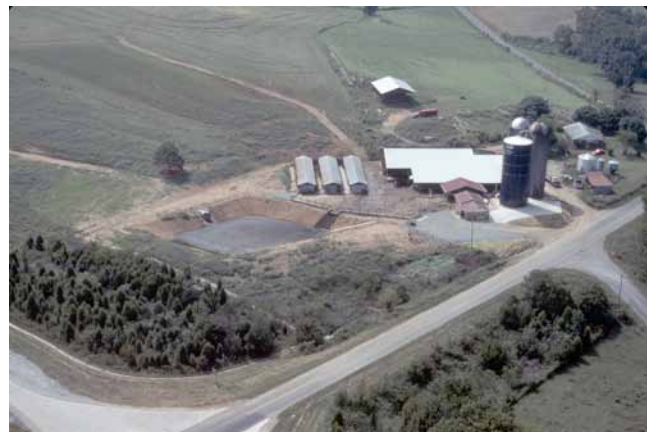
Figure 8–12 Vegetation near this recently constructed waste storage pond provides a screen.
