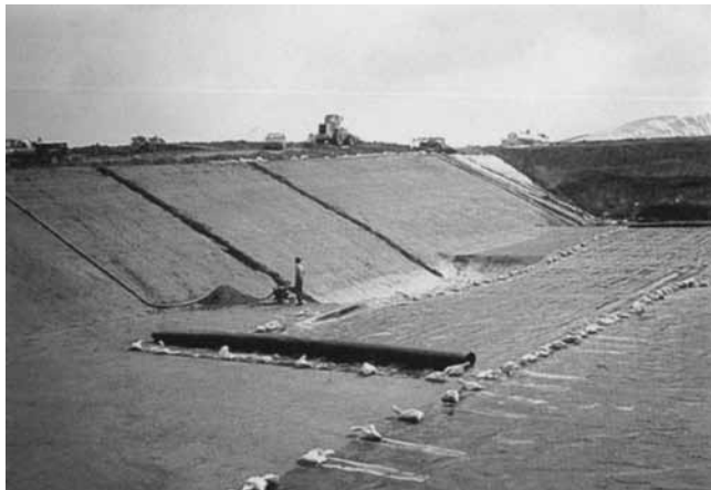
Figure 12–47 Membrane liner installation for earthen basin ( Photo and drawing courtesy of Hoechst Celanese Corp. )
