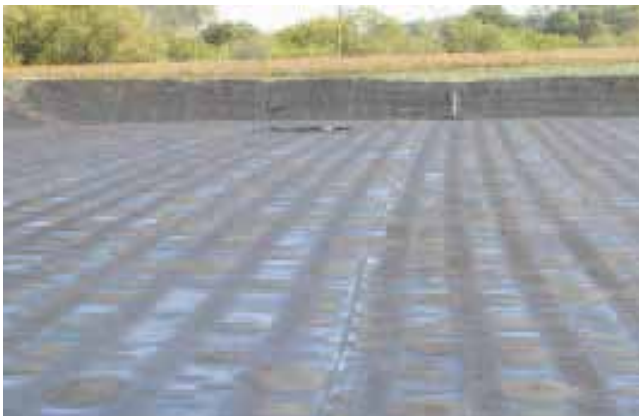
Figure 12-44 Closed-cell floating cover (Nicolai and Pohl 2004)
