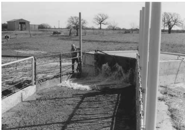
Figure 12–26 Hand-operated storage gate flush control (Photo courtesy of Agpro, Inc.)
