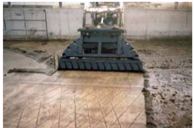
Figure 12-22 Grooved concrete to reduce slipperiness ( Photo courtesy of Mensch Mfg. )
