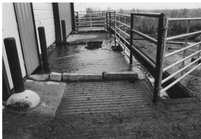
Figure 12–31 Cross gutter for alley flush water collection
