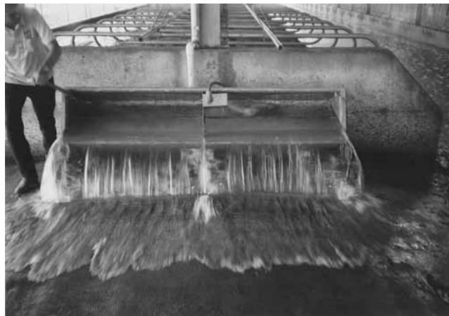
Figure 12–27 Flush water storage tank with dump-type release (Photo courtesy of Agpro, Inc.)
