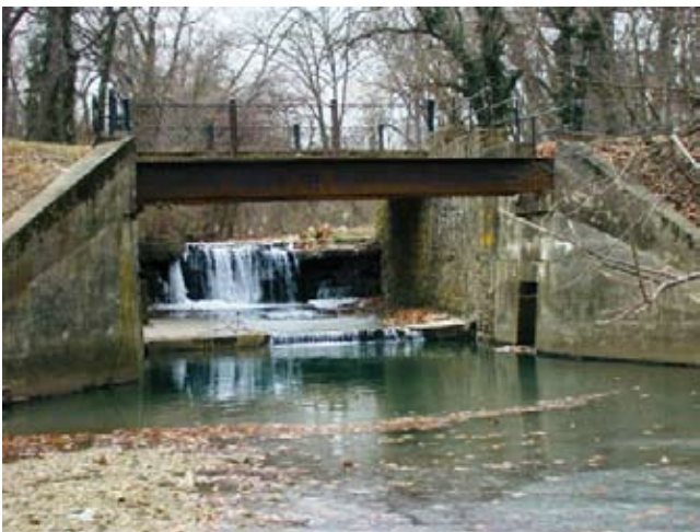
Figure 2-4 Fish blockage in stream
