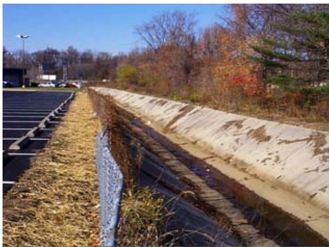
Figure 2-6 Stream encased by concrete channel
