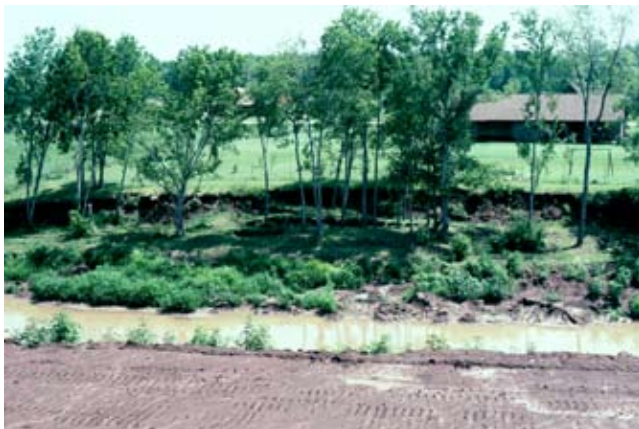
Figure TS14A-20 Stream slope that failed when the stream was deepened by about 4 feet to increase the flow capacity
