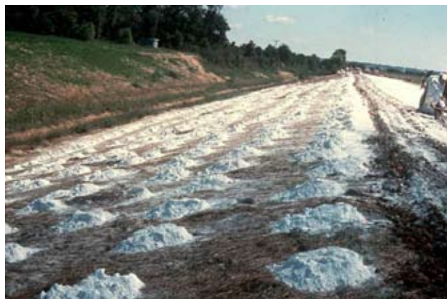
Figure TS14A-26 A streambank where highly dispersive clays were treated by applying and mixing in hydrated lime to the slope soils
