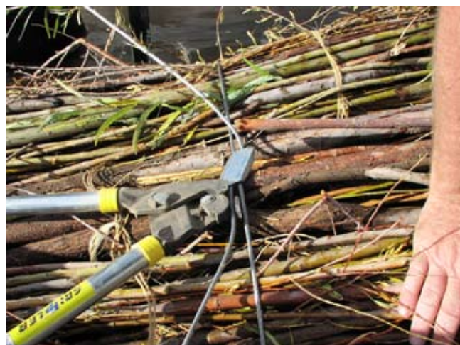
Figure TS14E-12 Gripple® wire rope grip and tensioning tool being used to tension down a brush spur
