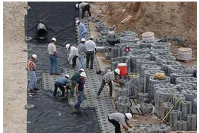
Figure TS14L-19 Hand placement of ACB blocks
