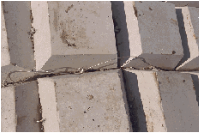
Figure TS14L-8 Steel cables
