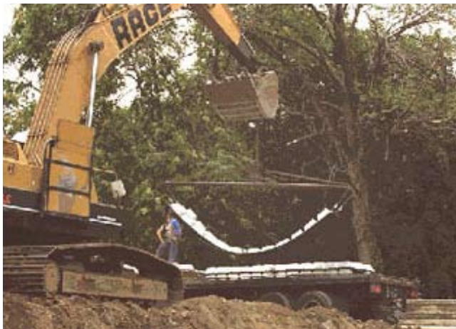
Figure TS14L-18 Spreader bar for placement of cabled mats
