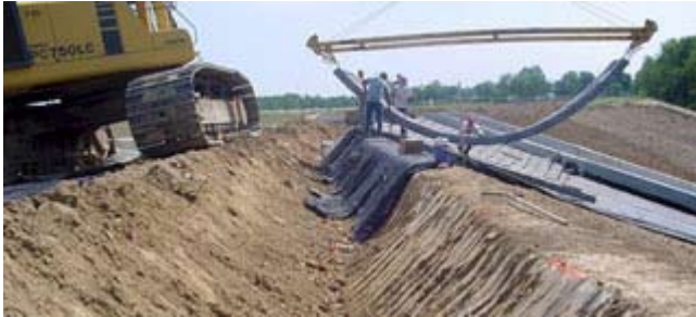
Figure TS14L-20 ACB termination trench
