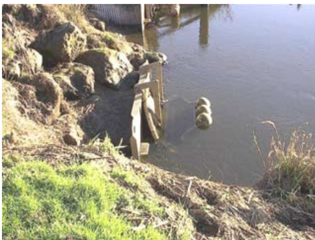
Figure TS14N-28 Self-regulating tide gate
