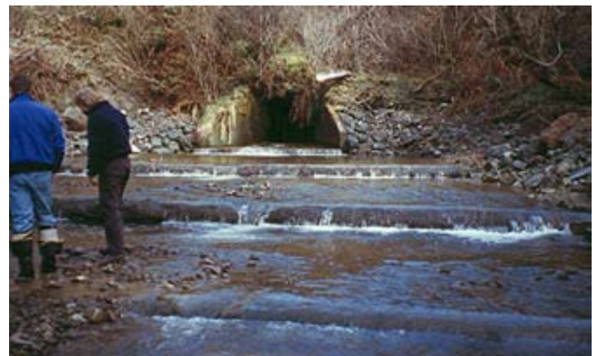
Figure TS14N-19 Series of channel spanning weirs used to step up water surface and raise outlet pool to culvert lip
