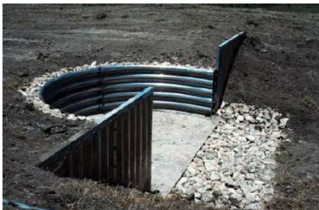
Figure TS14P-29 Grade stabilization structure
