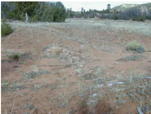
Figure TS14P-25 Rock and brush dam in AZ that has been working effectively ( Photo courtesy of Pete Bautista )
