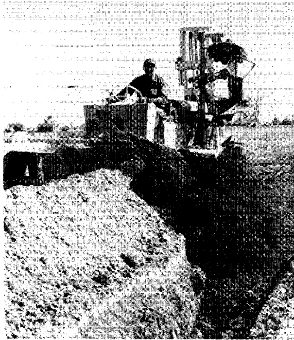
Backfilling with machinery
