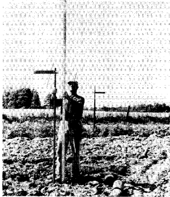
Setting targets for a trenching machine
