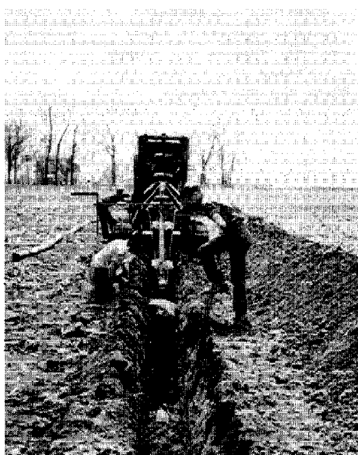
Blinding drain with a spade
