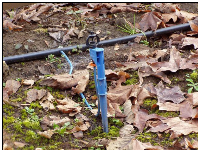
Figure SC6-29 Microsprayers suspended above ground on a spike fed by a feeder tube and polyethylene tubing
