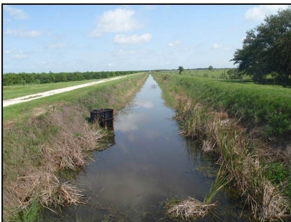
Figure SC6-41 A main ditch with a water table control structure to adjust depth of the water table in the field
