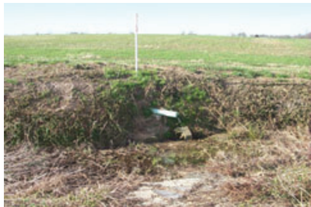
This outlet pipe is a sign of drain tile located in this field. Removal of drain tile is fairly simple, and outlets such as these are subsequently plugged.
