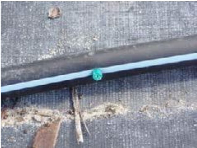
Figure 7–6 A microspray emitter with no moving part
