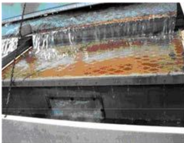
Figure 7–35 Water flowing over the screen in a gravity-flow filter
