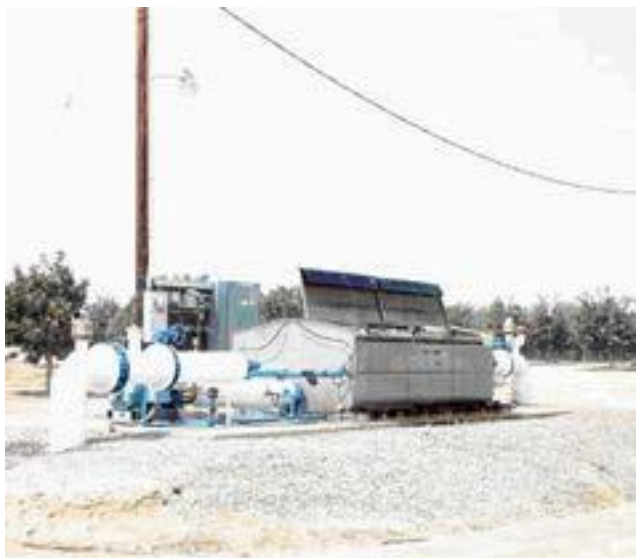
Figure 7–35 Water flowing over the screen in a gravity-flow filter
