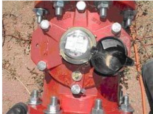
Figure 7-46 Typical in-line recording flowmeter
