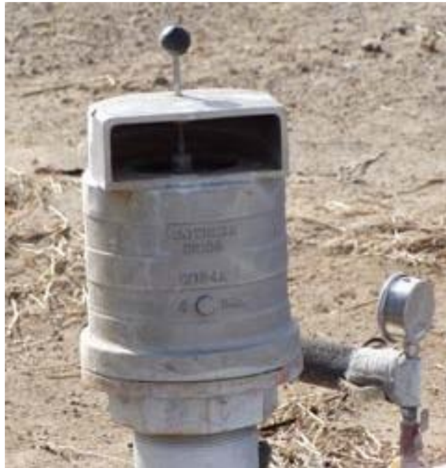
Figure 7-44 Combination air valve
