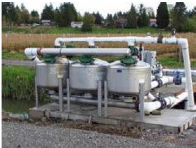
(c) A small, three-tank sand media filter
