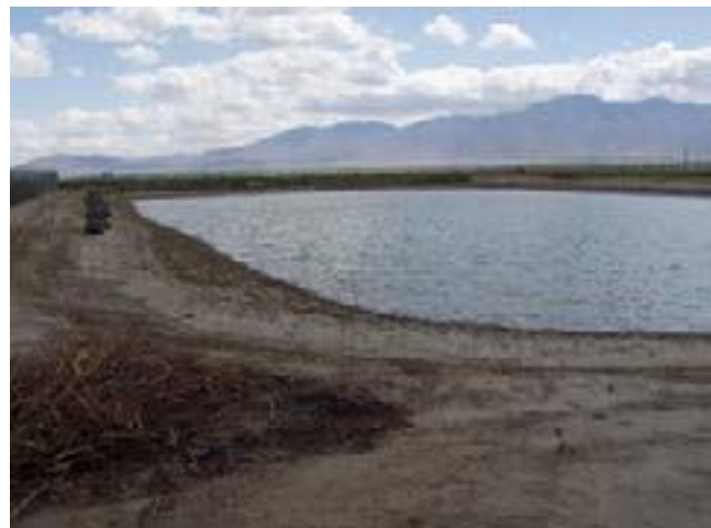
Figure 7–38 A well maintained settling basin
