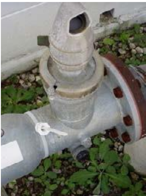
Figure 7–42 Air/vacuum relief valve
