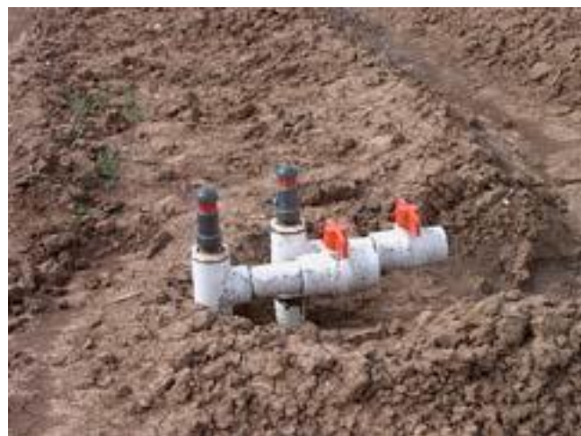
Figure 7–43 Automatic continuous acting air release valve
