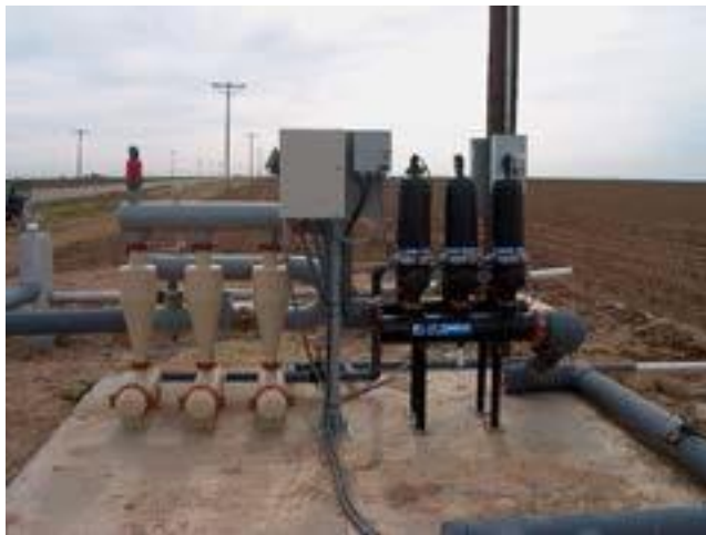
Figure 7–36 A three-unit vortex sand separator system (to the left of disk filters)
