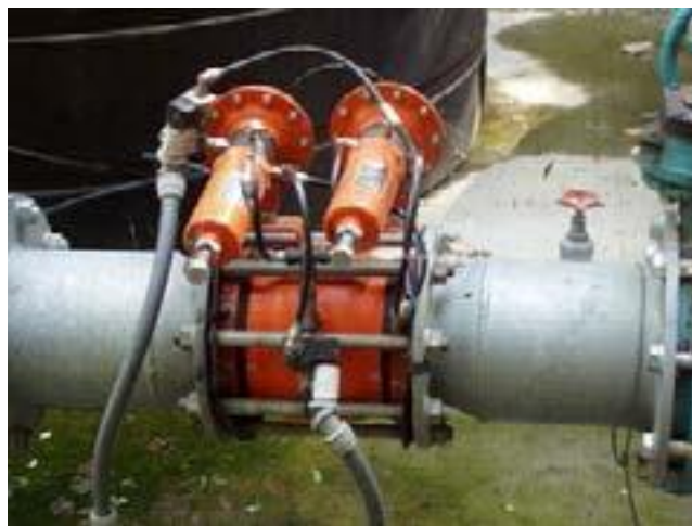
Figure 7–40 Solenoid controlled, pressure regulating valve
