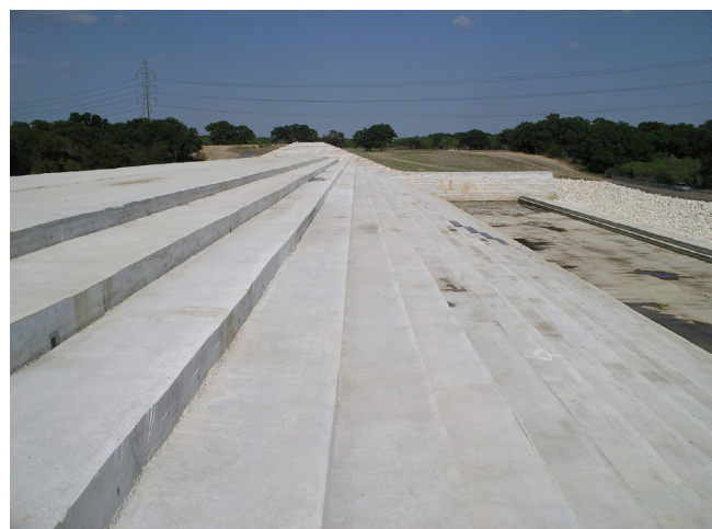
Figure 13–8 Finish that is uniform in appearance and relatively free from honeycomb and voids
