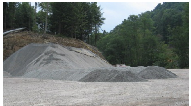
Figure 13–1 Keep pile height and steepness to a minimum to guard against segregation
