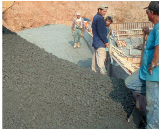
Figure 13–10 Mix piled against form
