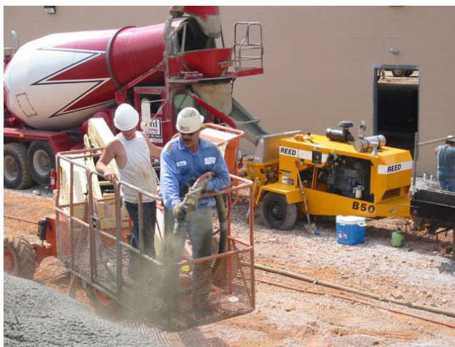
Figure 14-5 Concrete ready-mix truck discharging into concrete pump (Courtesy of REED Concrete Pumps & Shotcrete Equipment)
