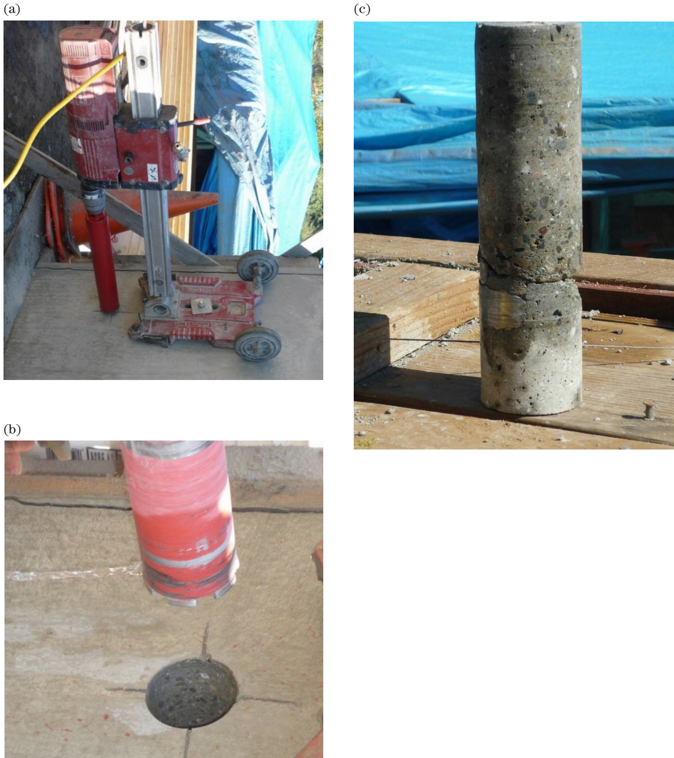
Figure 14–7 Coring test panels for compressive strength testing ( Courtesy of Bryan Mekechuk and Bill Brown )
