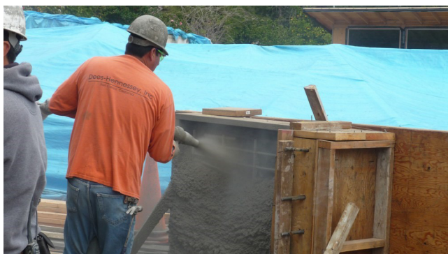
Figure 14–3 Nozzleman preparing a test panel (courtesy of Bryan Mekechuk and Bill Brown)
