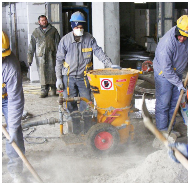
Figure 14–4 Workers loading premixed dry components into a shotcrete gun (Courtesy of REED Concrete Pumps & Shotcrete Equipment)
