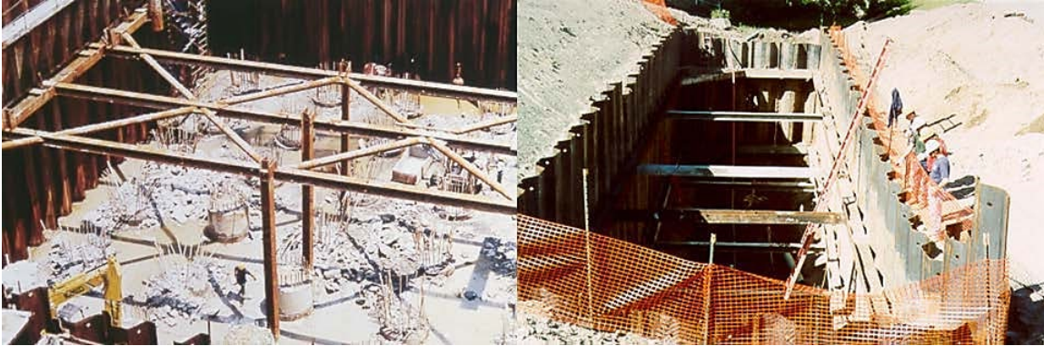
Figure 645R-28. Example of Steel Sheet Piling with Bracing (NRCS)
