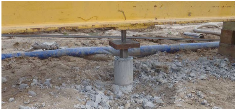
Figure 645R-10. Typical Installed Micropile (NRCS-OK)
