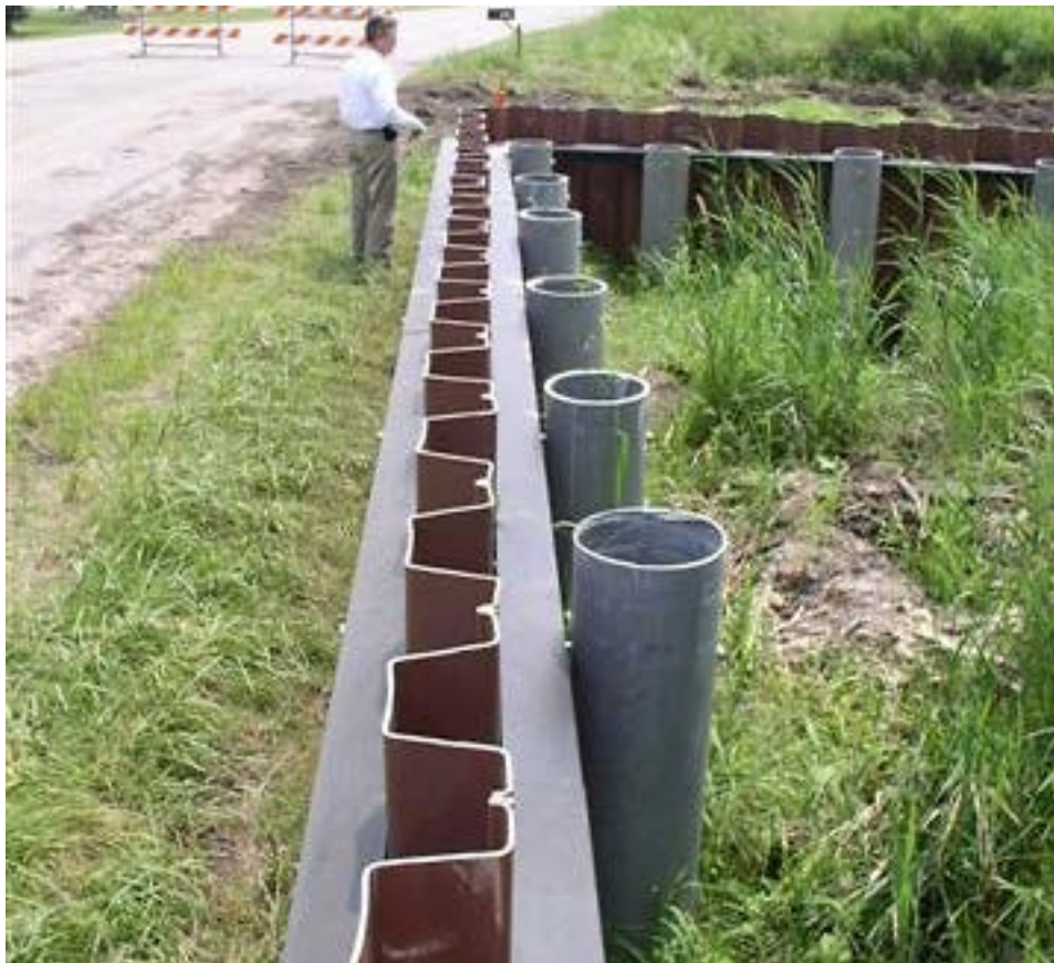
Figure 645R-30. Vinyl Sheet Pile with Walers and Soldier Piles
