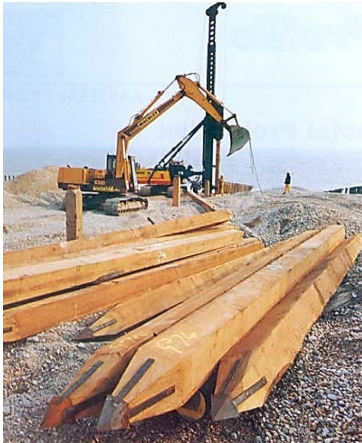
Figure 645R-5. Timber Piles with Steel Points on the Tips (USDA)
