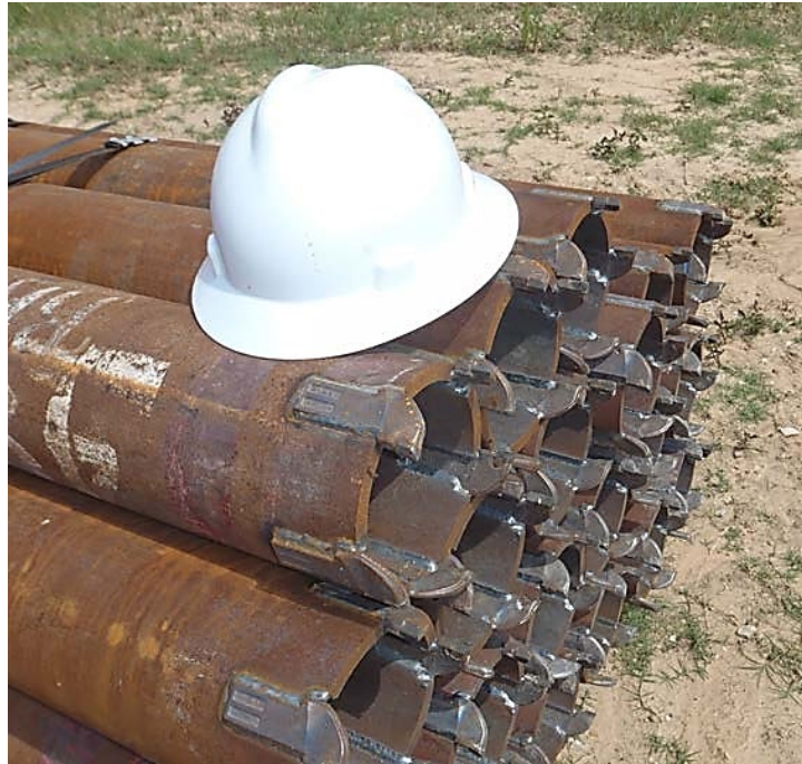
Figure 645R-12. Micropile Casing (NRCS-OK)
