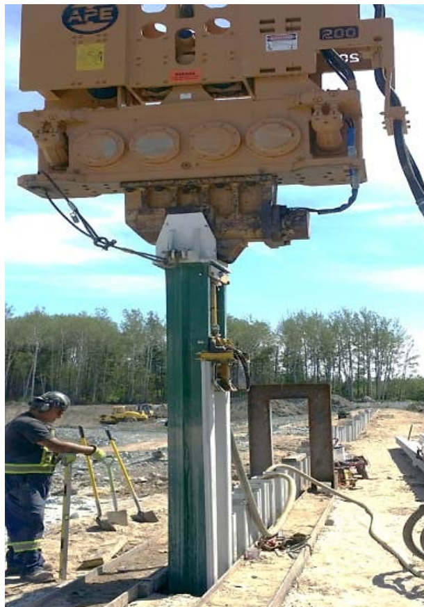
Figure 645R-29. Installation of Vinyl Sheet Pile with Mandrel (Wolf Remediation, Ltd.)
