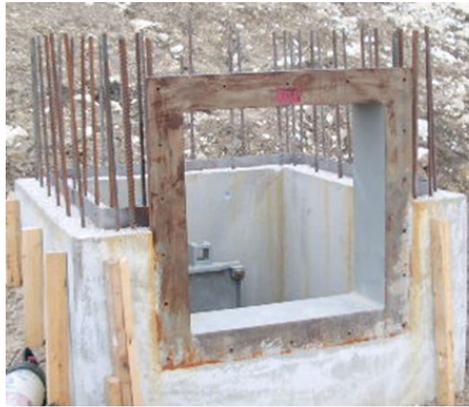
Figure 645S-7: Wall Thimble (NRCS TX)
