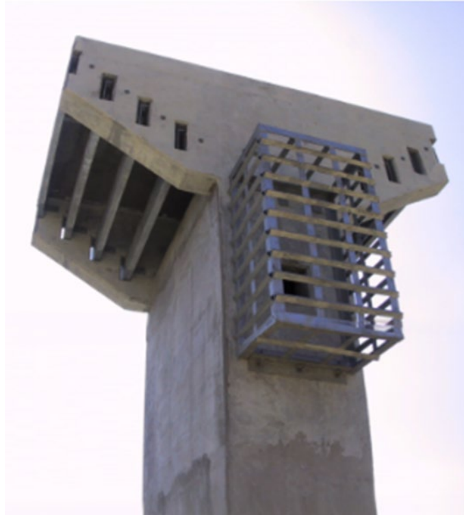
Figure 645S-11: Metal Baffles and Trash Rack Assembly (source: NRCS OK)
